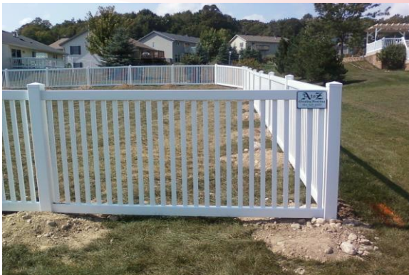
DJ 2 - 4' flat top open picket with 2" spacing
