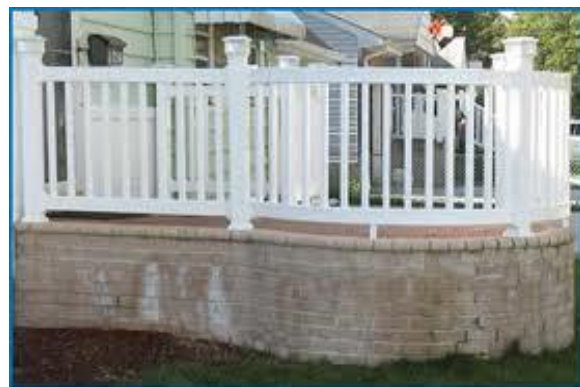
DJ 3 - 4' flat top open picket with 3" spacing
